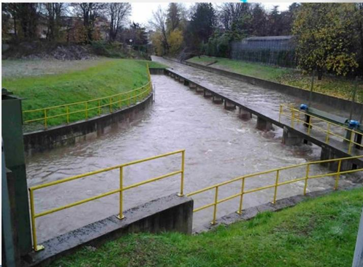
Bypass channel (CSNO, acronym from Italian “Canale Scolmatore di Nord Ovest”). Built from 1954 to 1980. Discharge capacity 30 m<sup>3</sup>/s
